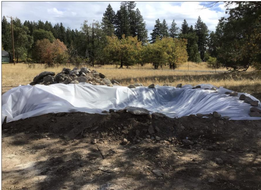
Photo 2: The concrete washout was re-lined prior to use.
