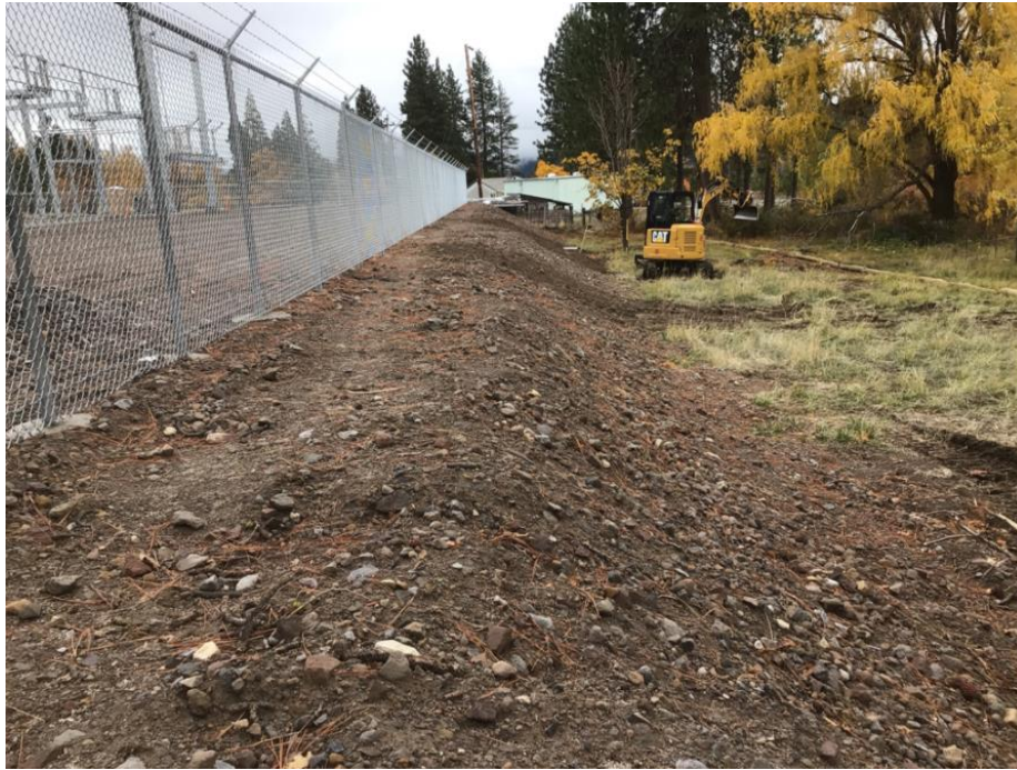
Photo 3: Operator restoring the west side of the substation.
